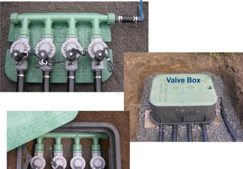
The sprinkler wire needs to have at least one more wire strand than the number of valves being installed
